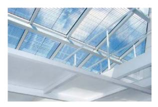
the adhesion of the glass to the interlayer means that laminated glass, even when broken, tends to remain in place, protecting occupants and property from injury and damage caused by rain, wind, snow, etc.
