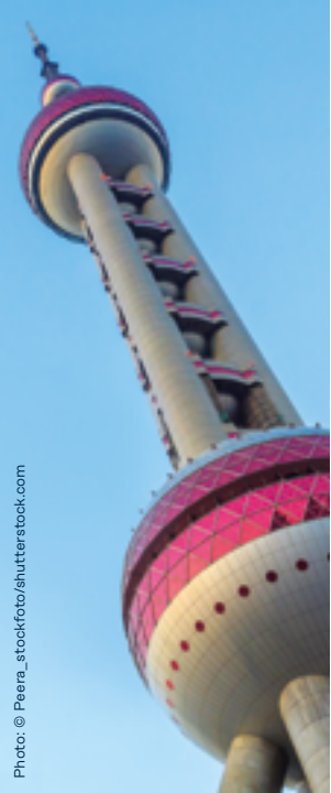
Shanghai Pearl Tower, China
