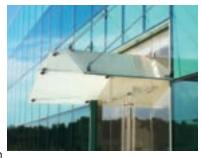
exposed edges (canopies, handrails and pointsupported walls). SentryGlas® is available in .035, .060, and .090 thicknesses.
