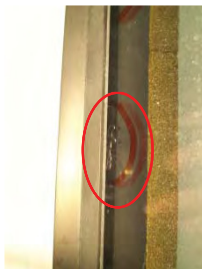
Figure 9: "Delamination" in sample 44.2-HA-B/07, after 7 weeks UV irradiation test
