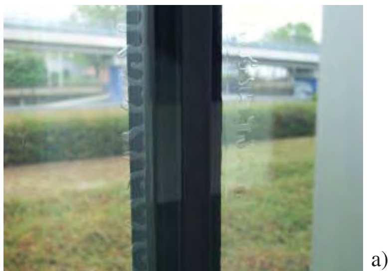
Figure 14 - Defect in IGU with laminated glass pane: a) defect starting from the glass pane edge; b) defect starting from a bubble
